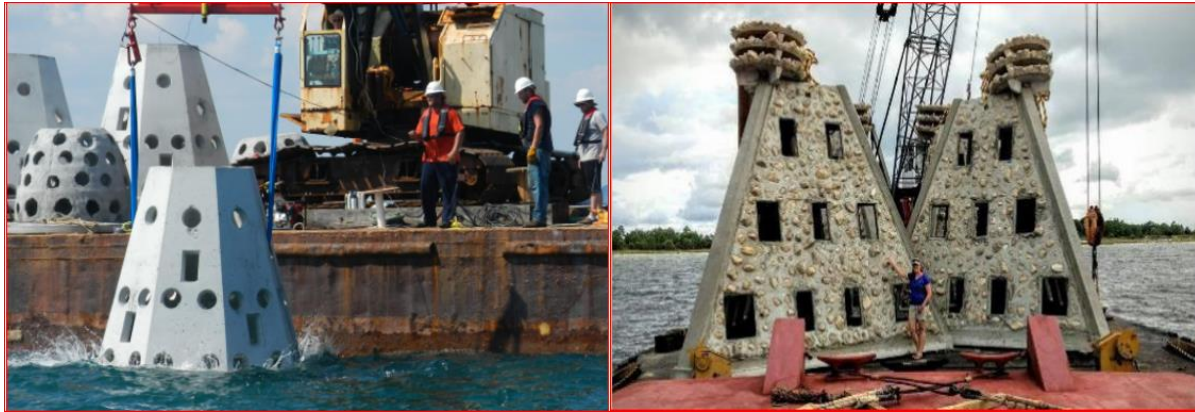
Pic. N4 Artificial Reef - Massive Cement Construction (3-5 m. Height)
